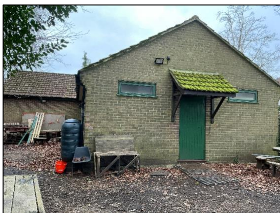
Photograph 10. Northern aspect of B1
