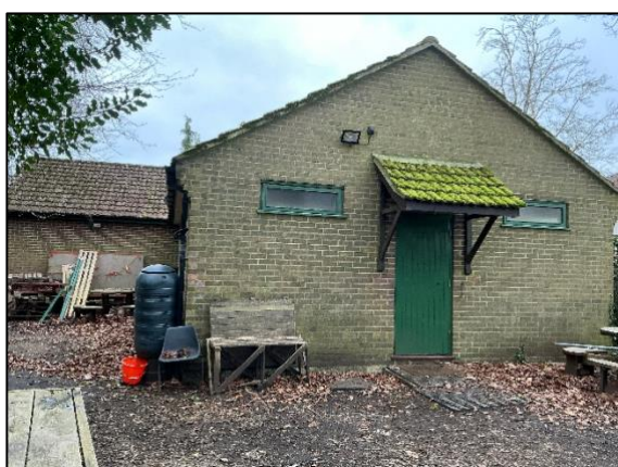
Photograph 5. Northern aspect of B1
