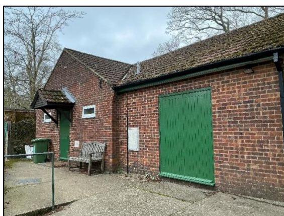
Photograph 6. Southern aspect of B1
