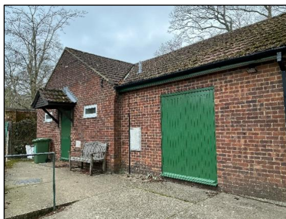
Photograph 11. Southern aspect of B1
