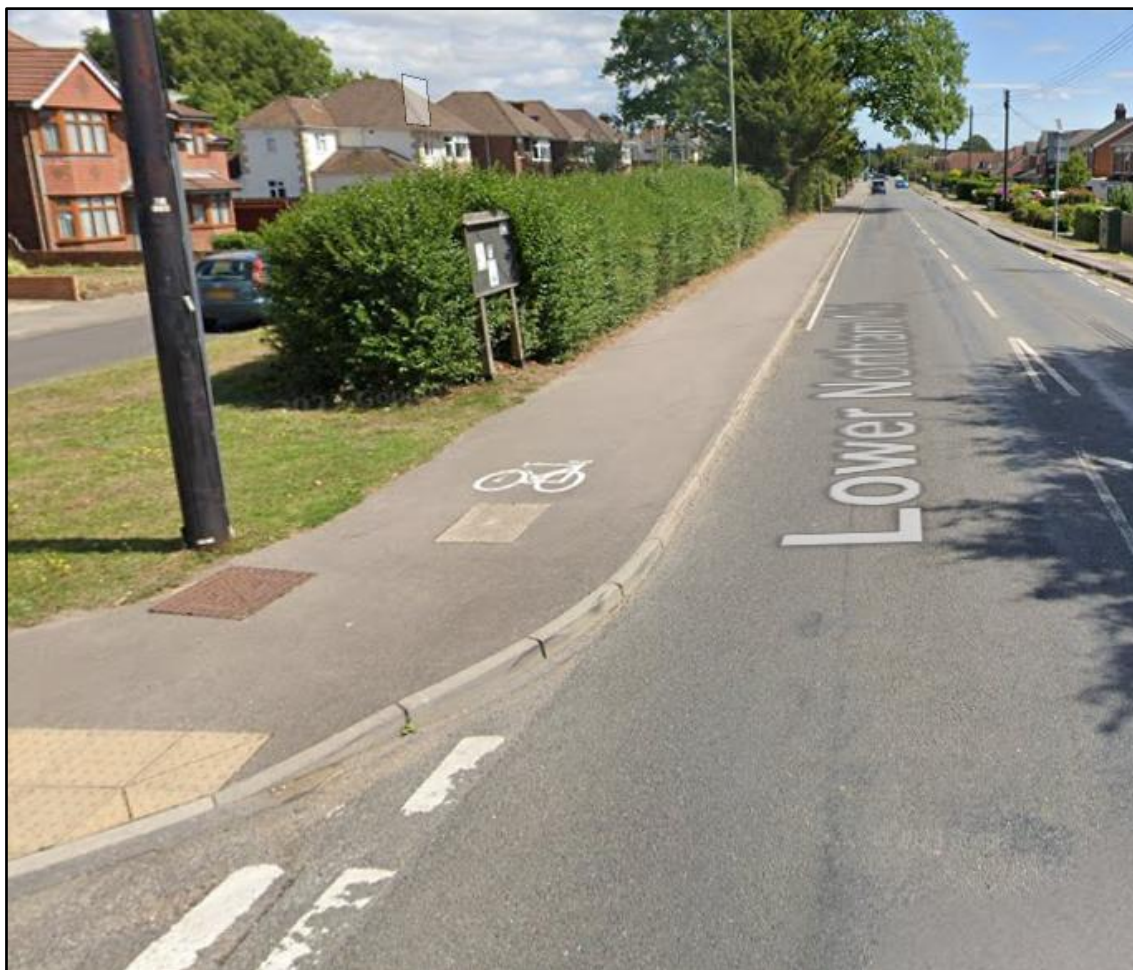
Image 3.4: Lower Northam Road – Shared use footway / cycleway.
