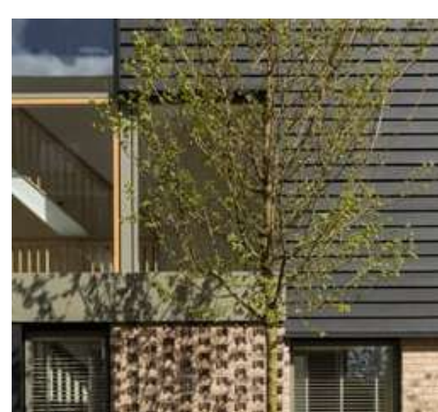
Contrasting brick / vertical boarding.
