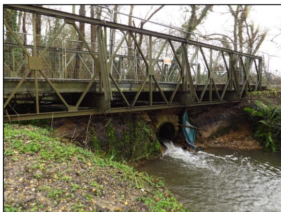
Photo 7 Southern extent of the bridge
