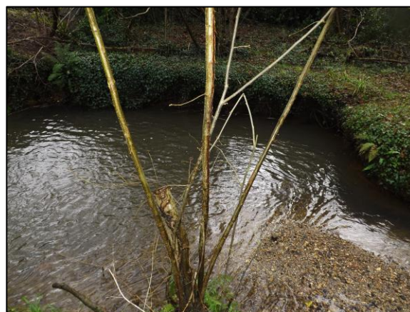
Photo 8 Large pool after the water flows through the culvert.
