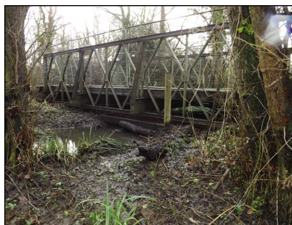
Photo 6 Northern extent of the bridge
