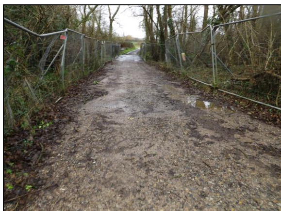
Photo 3 Existing haul road comprises a gravel track
