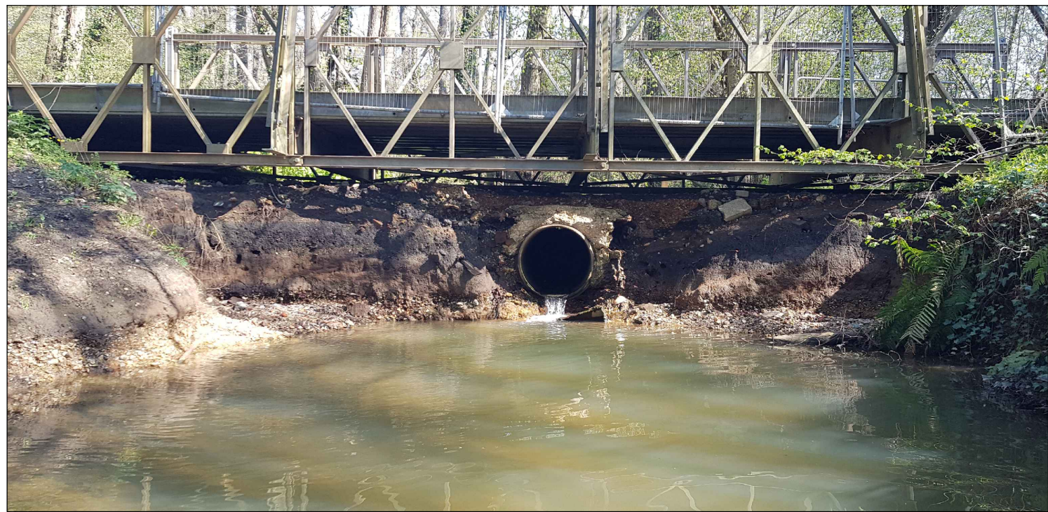
PHOTO OF EXISTING DOWNSTREAM STRUCTURE
