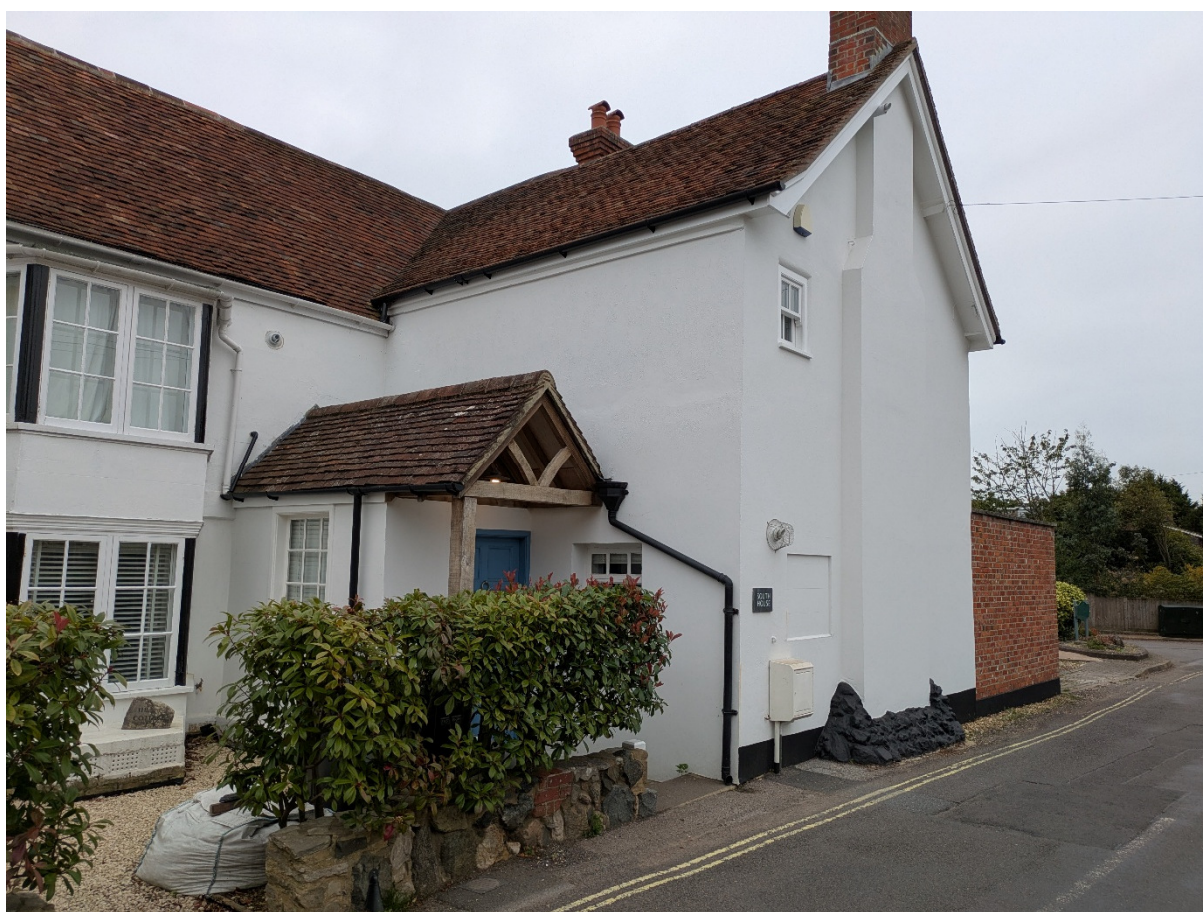
Street-level view of South House from the North-West
