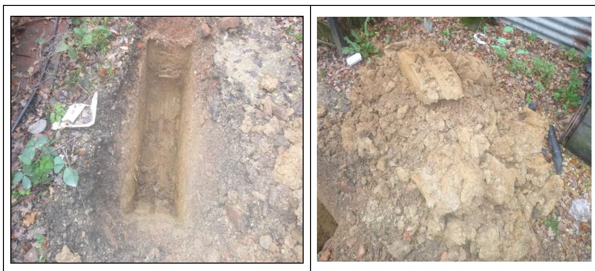
Photograph 1 Trial pit and removed soil material - Location TP.01
