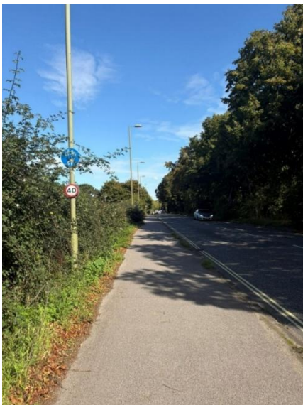
Figure 19: Footway / Cycleway along A335 Wide Lane
