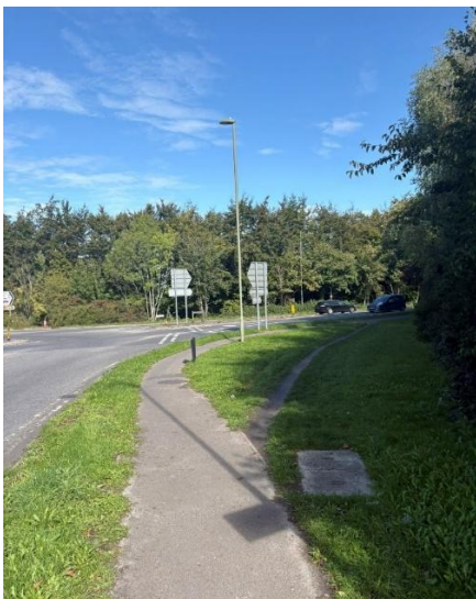
Figure 16: Footway / Cycleway at the A335 / Wide Lane Roundabout
