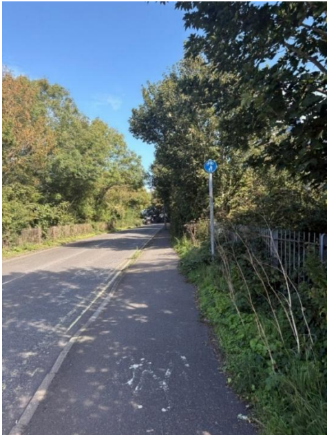
Figure 14: Wide Lane Footway / Cycleway
