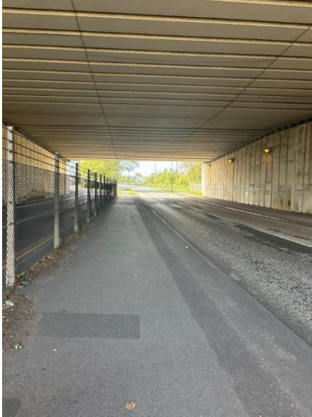
Figure 43: Wide Lane Tunnel Under M27
