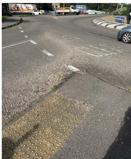
Figure 42: George Curl Way Loose Gravel and Overgrown Vegetation on Wide Lane (W) Crossing
