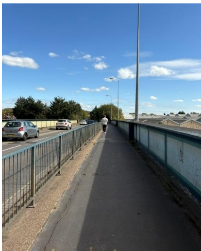
Figure 39: Bishopstoke Road Bridge Footway / Cycleway
