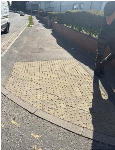
Figure 30: Chickenhall Lane Tactile Paving
