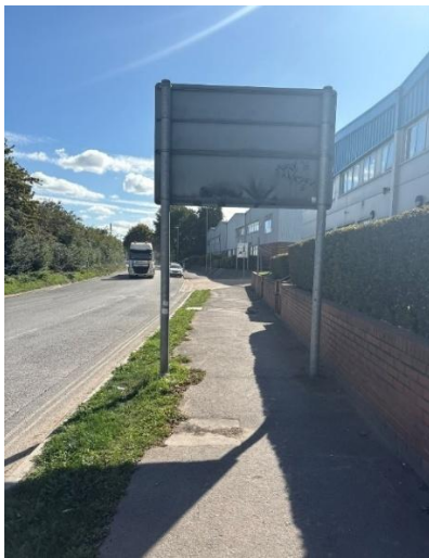
Figure 32: Furniture and Utilities within Footway
