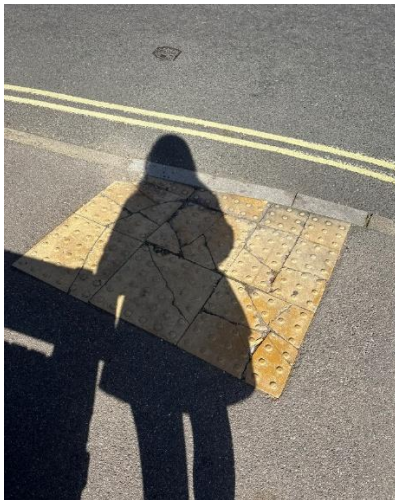
Figure 24: Derby Road Tactile Paving
