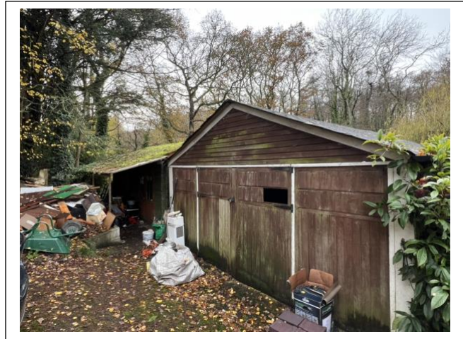
Existing outbuildings to be removed
