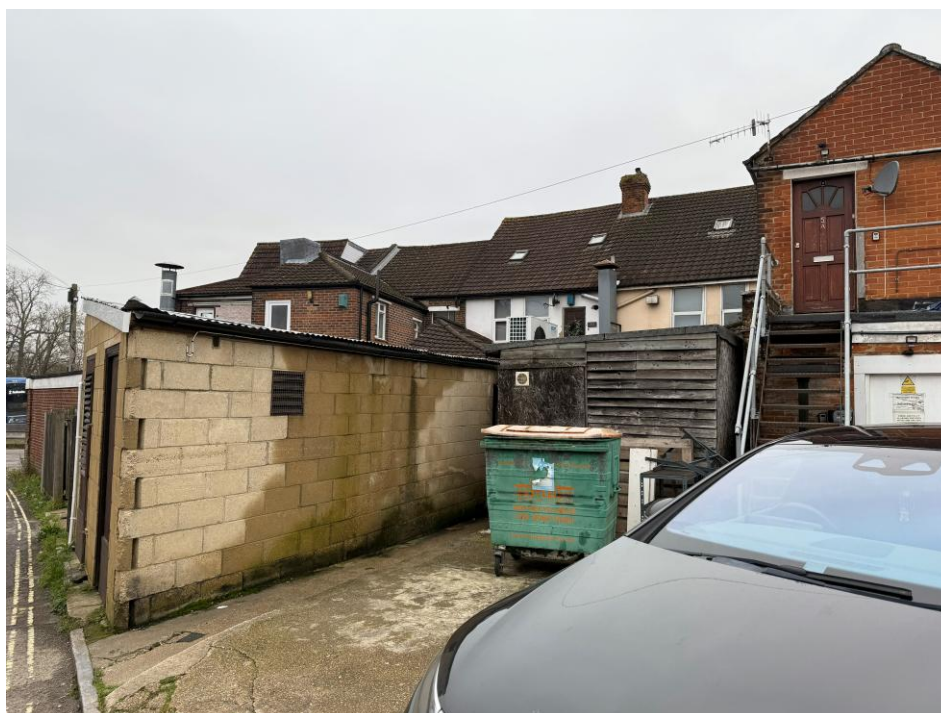
Figure 4 - Photograph of the rear from Montague Road
