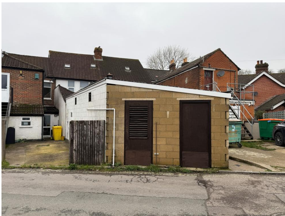
Figure 3 - Photograph of the rear from Montague Road
