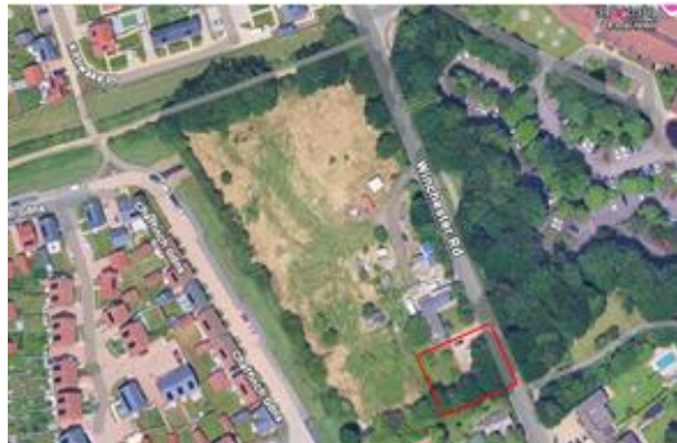
Image 2: Aerial view of the site
