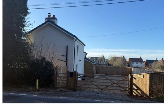
Image 15: Oak cottage to the north with new development Beyond
