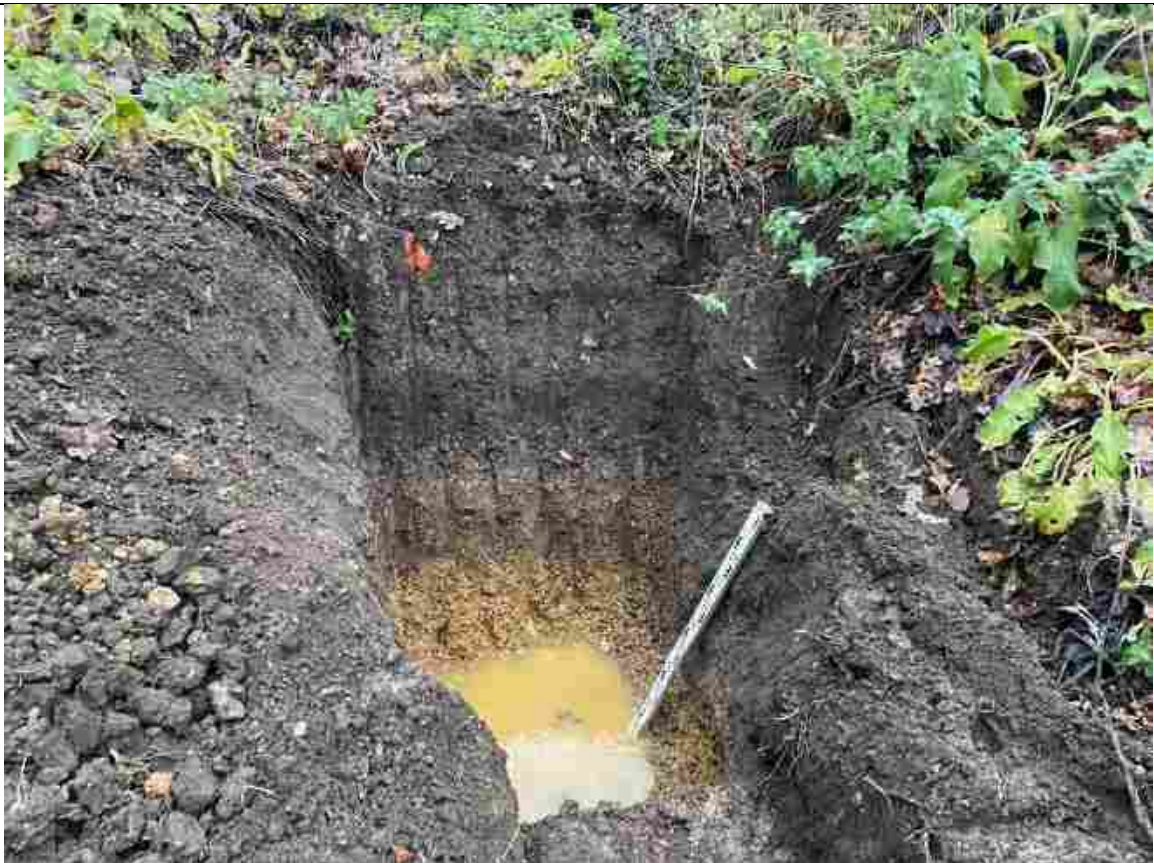
PLATE 2 – Water at base of trial pit at c.0.9m where the 300x300mm sumps would have been dug
