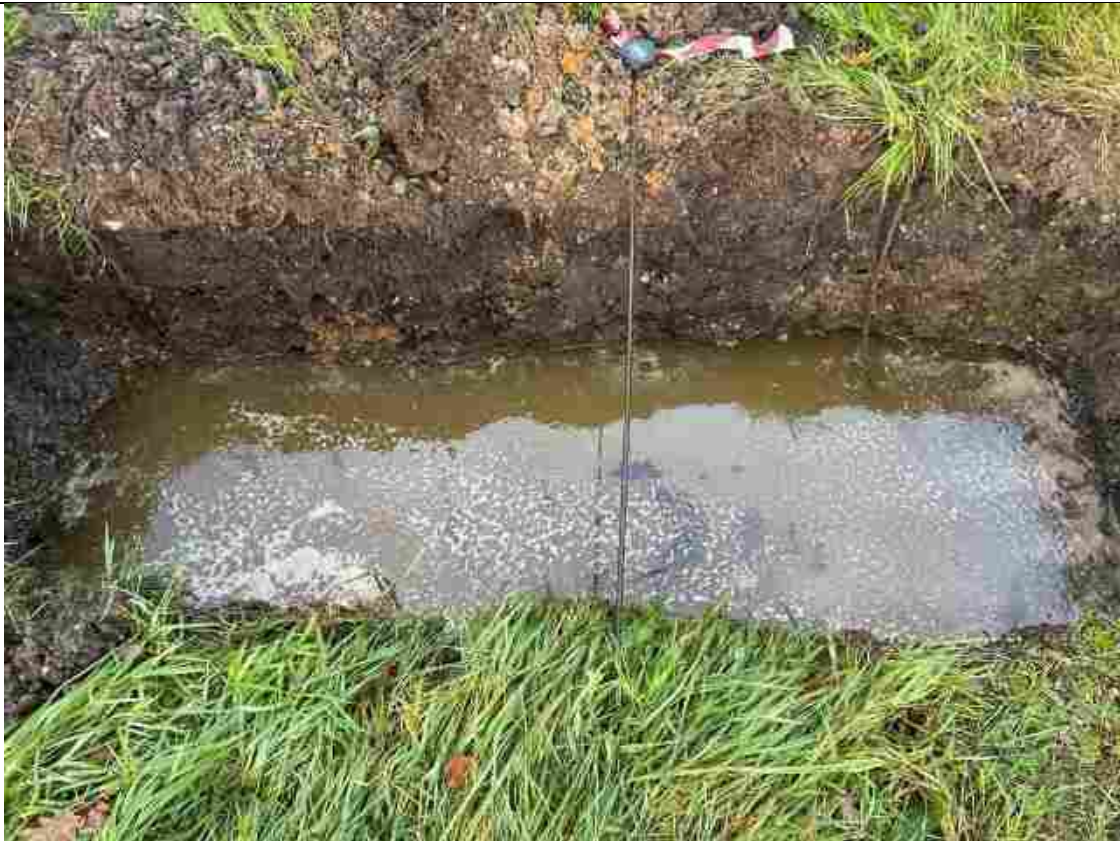
PLATE 23 – Standing water level in Structure 6 trial pit at start of the infiltration test
