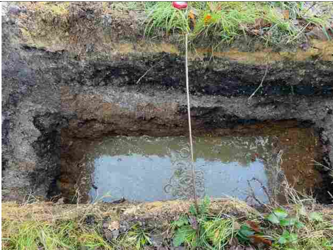
PLATE 25 – Standing water level in Structure 7 trial pit at start of the infiltration test
