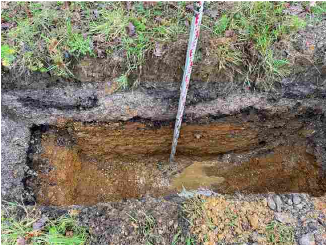
PLATE 14 – Structure 2 trial pit
