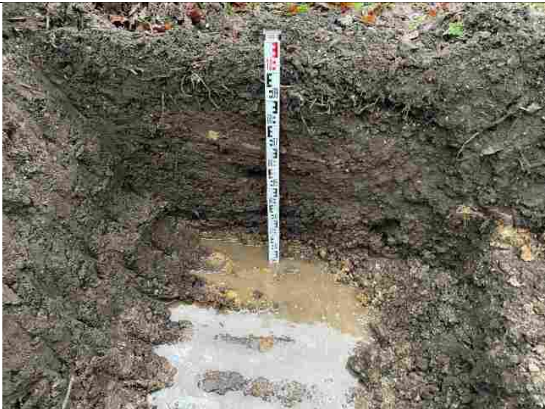
PLATE 7 – Water entered the trial pit during excavation
