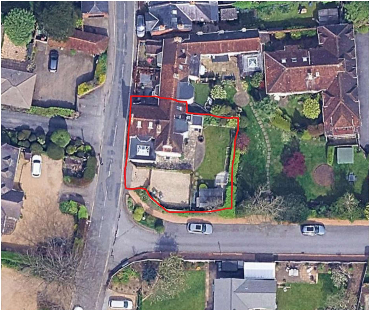
Aerial view of the site with the boundary shown in red
