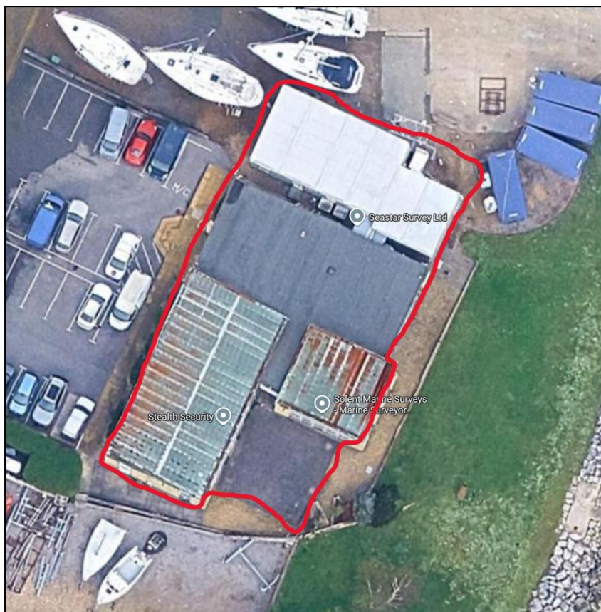
Figure 1: Building to be demolished.
