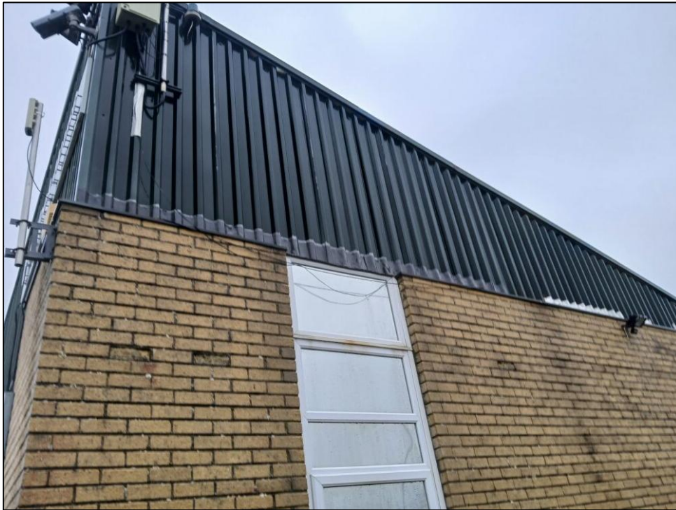
Photo 1: Building B1, southern aspect
