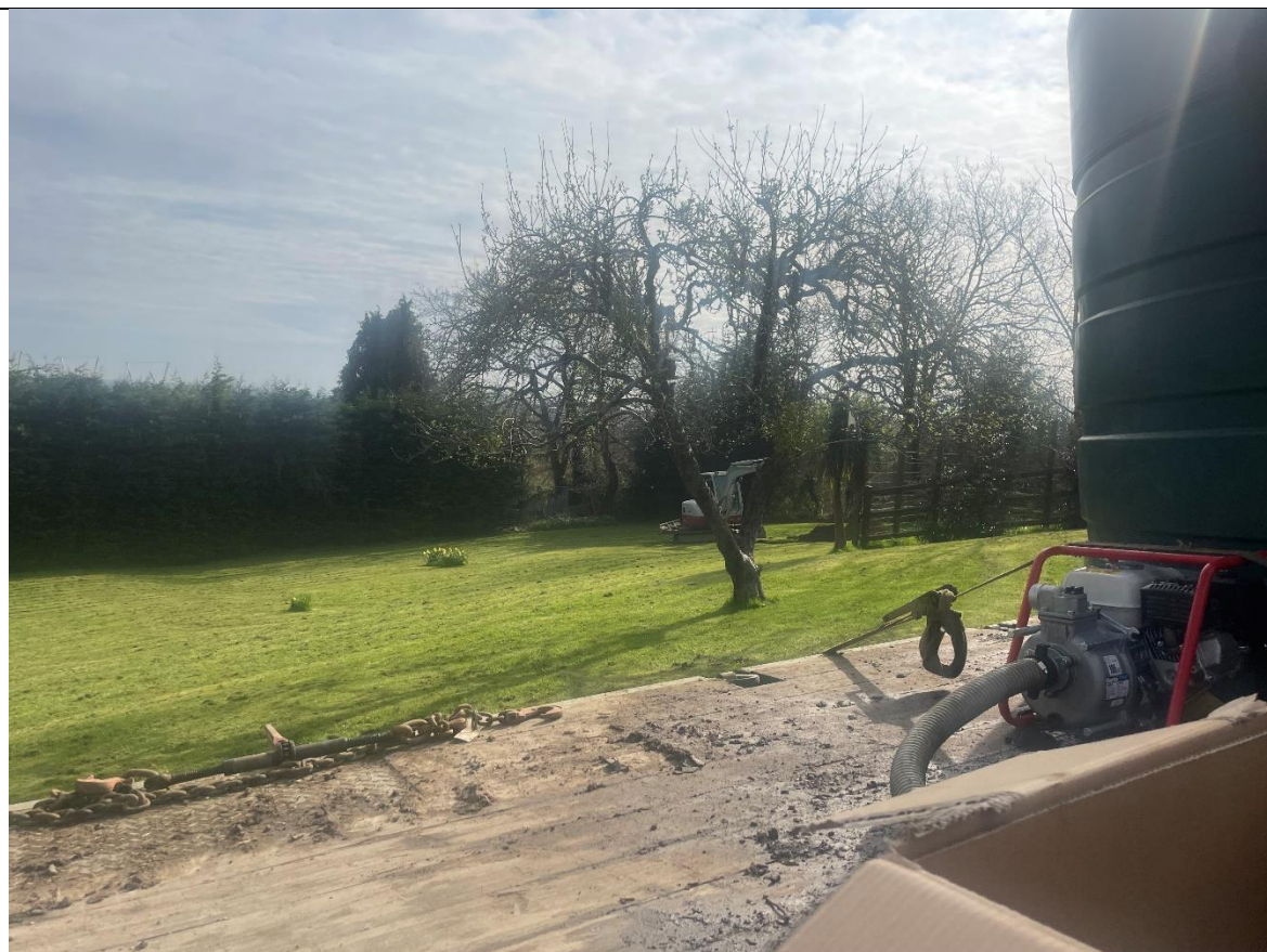
PLATE 2 – Digging test pit SA02
