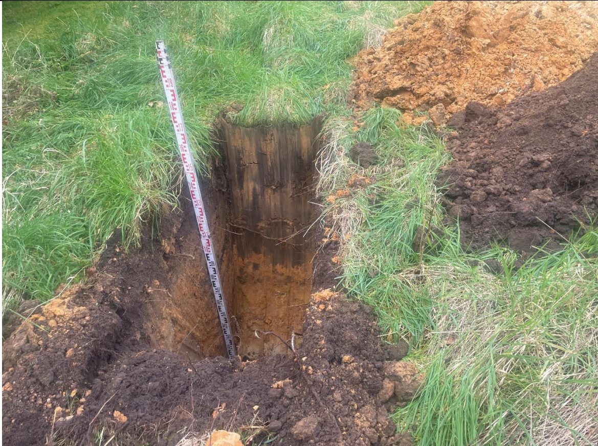
PLATE 1 – Infiltration Test Pit SA01 and arisings
