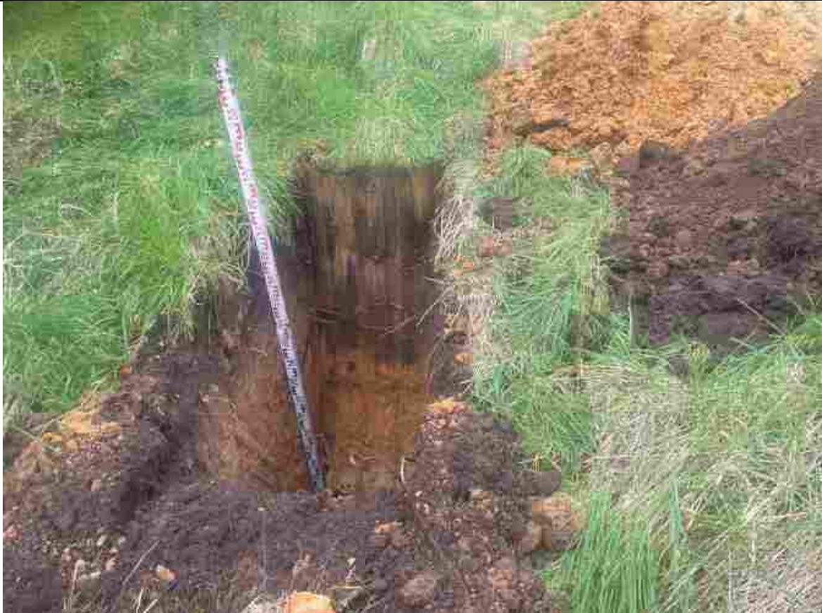
PLATE 1 – Infiltration Test Pit SA01 and arisings
