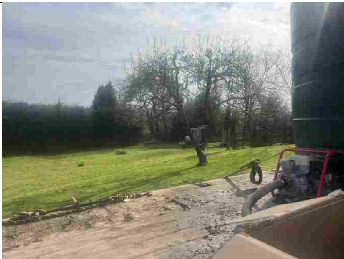
PLATE 2 – Digging test pit SA02
