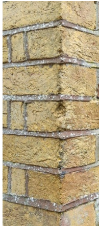
Figure 3-Existing brick to be matched for rear extension
