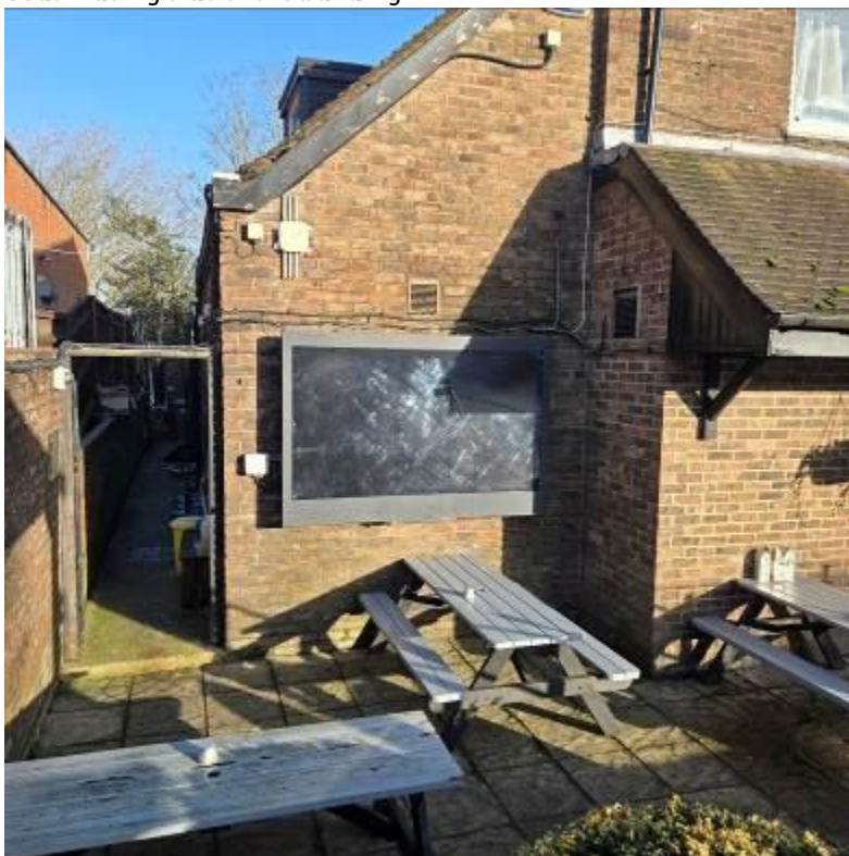
Photograph showing position of installed TV on the building, which is set back from the foreground elevation to the South facing side of the building.
