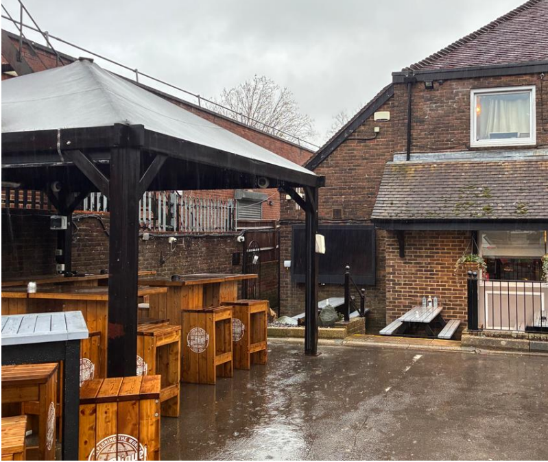
Photograph showing position of installed TV on the building, which is set back from the foreground elevation to the South facing side of the building.
