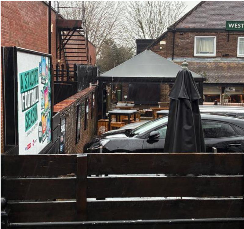
Photograph showing position of installed TV on the building, which is set back from the foreground elevation to the South facing side of the building. The fence and surrounding walls obstruct the view from the roadside.
