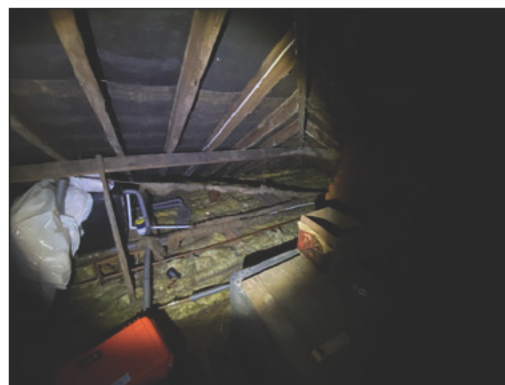
Figure 4 – Interior roof void of the main house.
