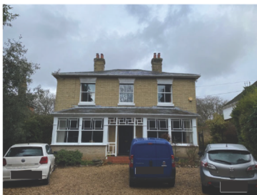
Figure 1 – Southern elevation of the dwelling.
