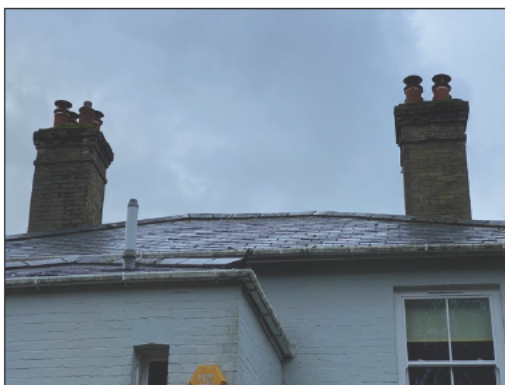
Figure 3 – Northern slate roof of the main house.
