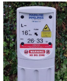
Mainline marker post
