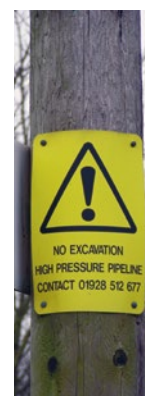
Pole warning marker
