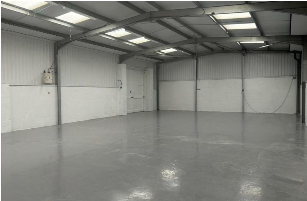
Figure 11 – Internal refurbishment of resin floor.
