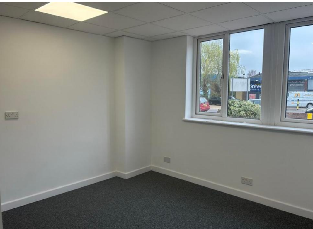
Figure 12 – Internal refurbishment (front office)
