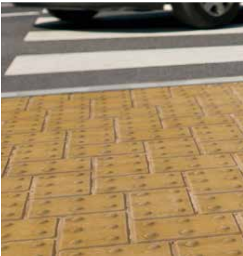
Tactile Paving Marshalls - Blister paving (or similar)
