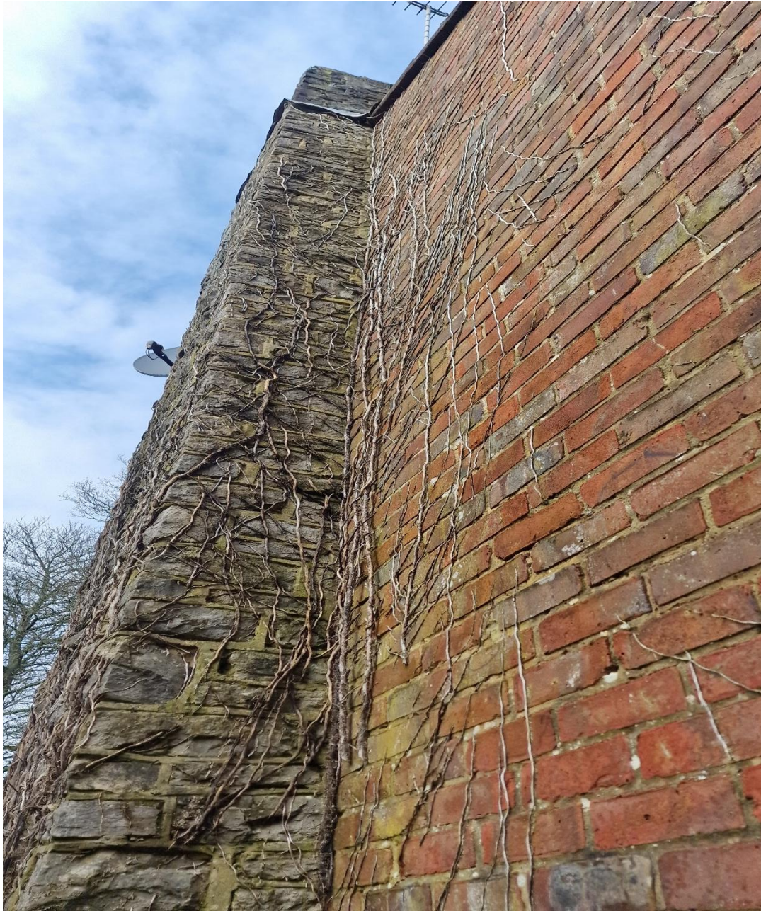
Picture 3: Showing the southern gable wall
