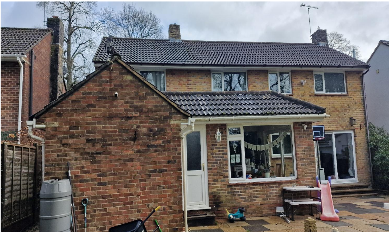
Picture 2: Showing the rear elevation
