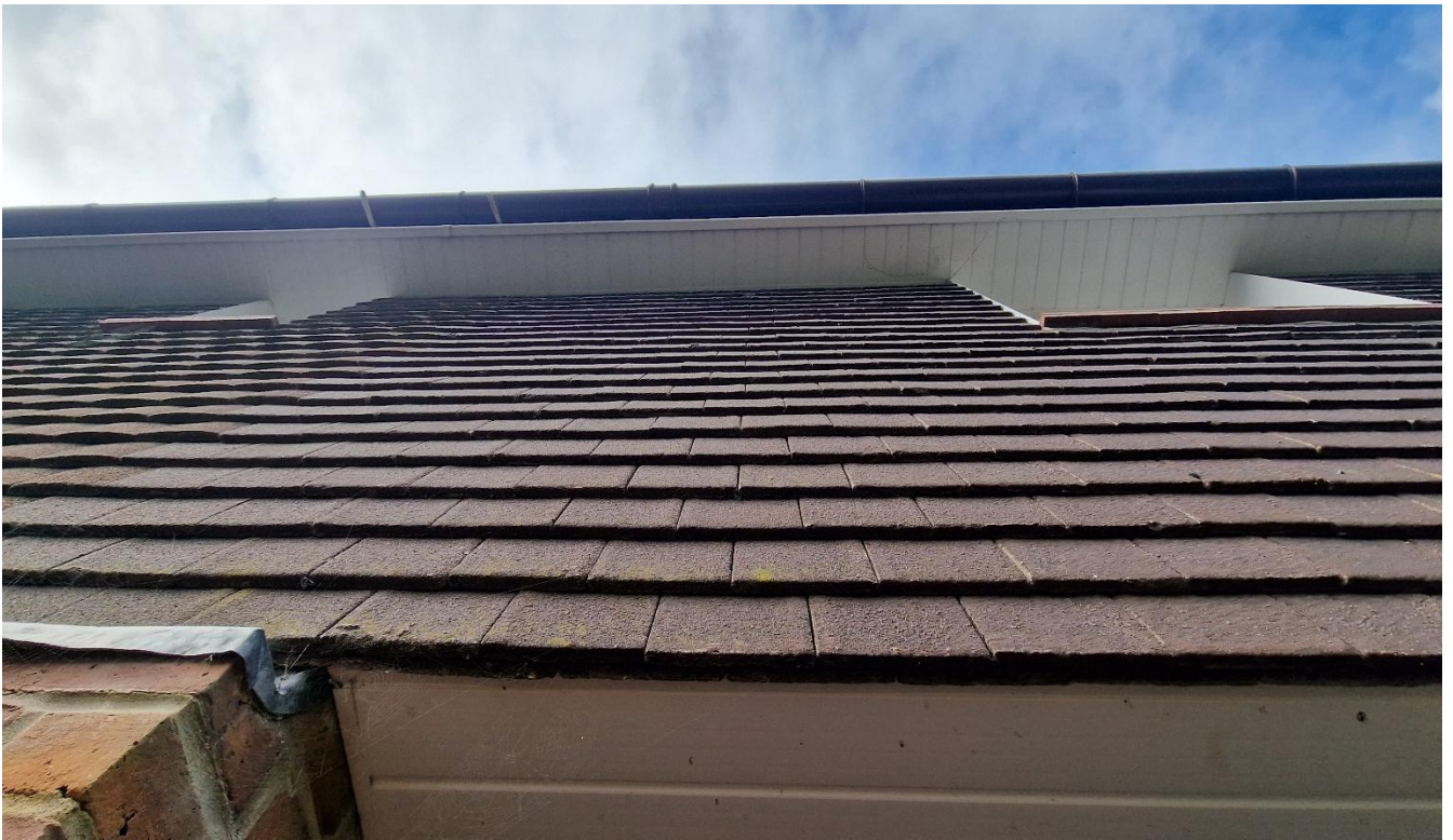
Picture 5: Showing tight fitting tile hanging
