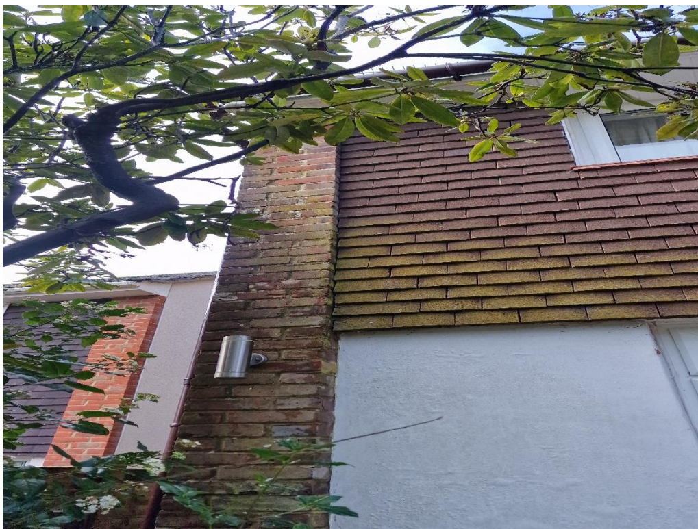
Picture 7: Showing the area where the tile hanging meets the wall, no gaps or holes
