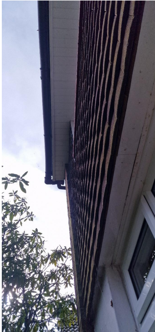
Picture 11: Showing tight fitting tile hanging and UPVC eaves
