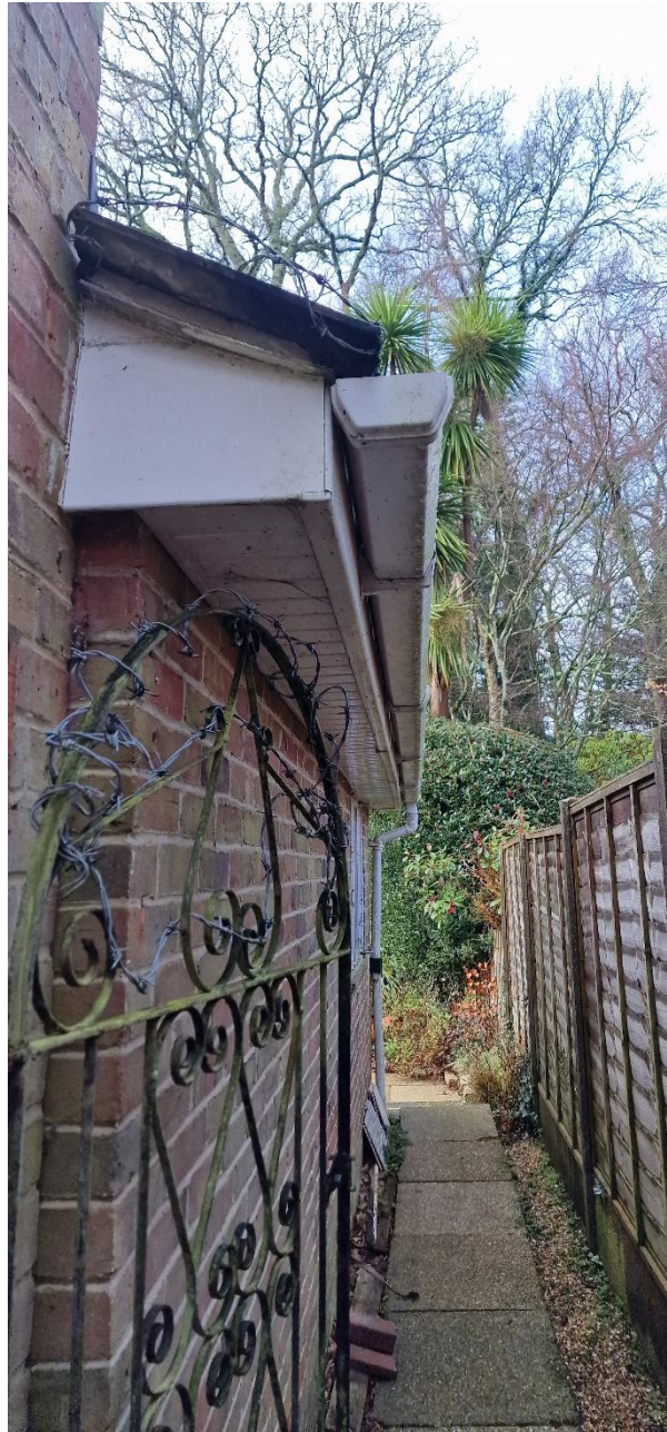
Pictures 10 : Showing the eaves of the single storey extension
