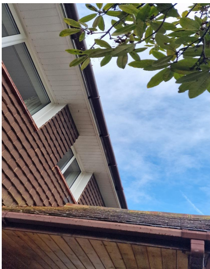
Picture 8: Showing the tiles over the porch, upvc eaves
